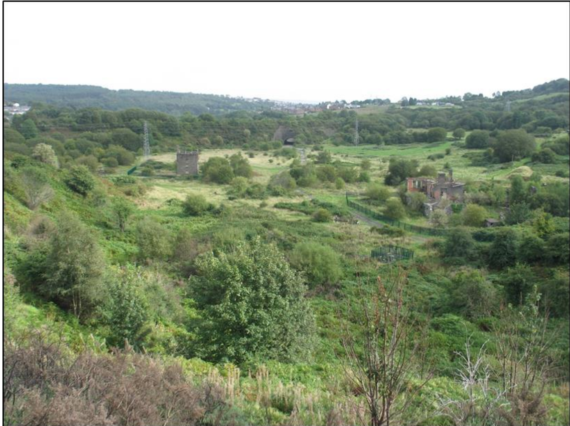
The British (Abersychan) Ironworks Site with scheduled/listed Engine House, left and listed Office and Workshop Quadrangle, right (© Glamorgan-Gwent Archaeological Trust and Cadw)
